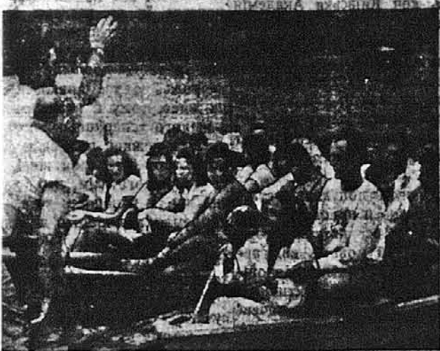
STUDENTS at the American Red Cross aquatic school at Camp Carolina, Brevard, N. C., learn to "make a disaster" calamaran by taping three boats together. On boards placed across the gunwales, 32 people may be carried instead of the normal complement of six to a boat. (American Red Cross Photo)
